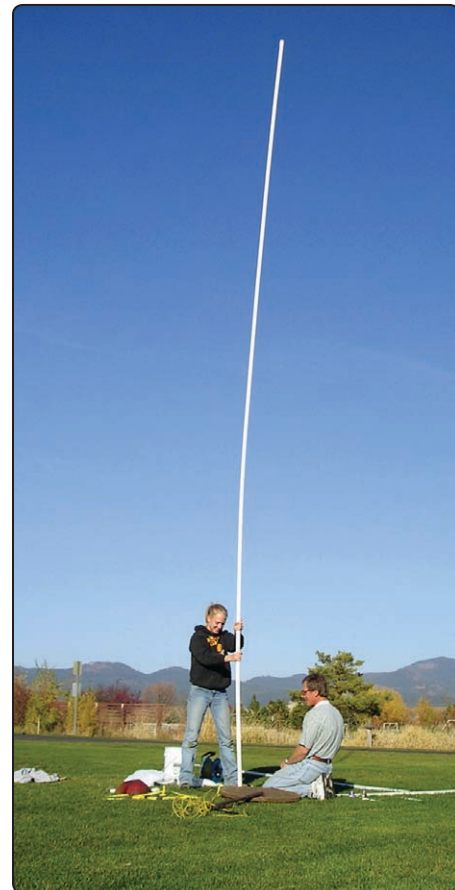
Installing Instrumentation Guide Tube in Monitoring Well
