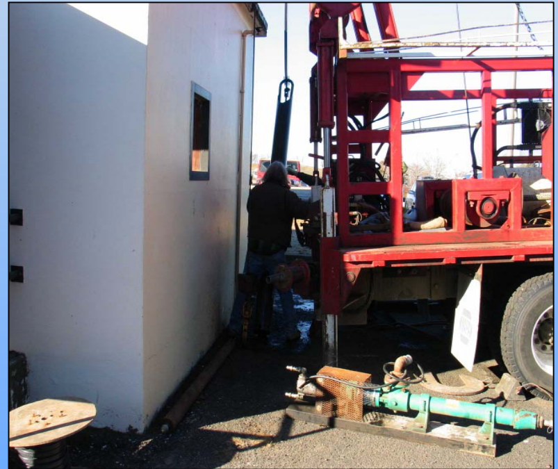
Driller preparing bailer to dump.
