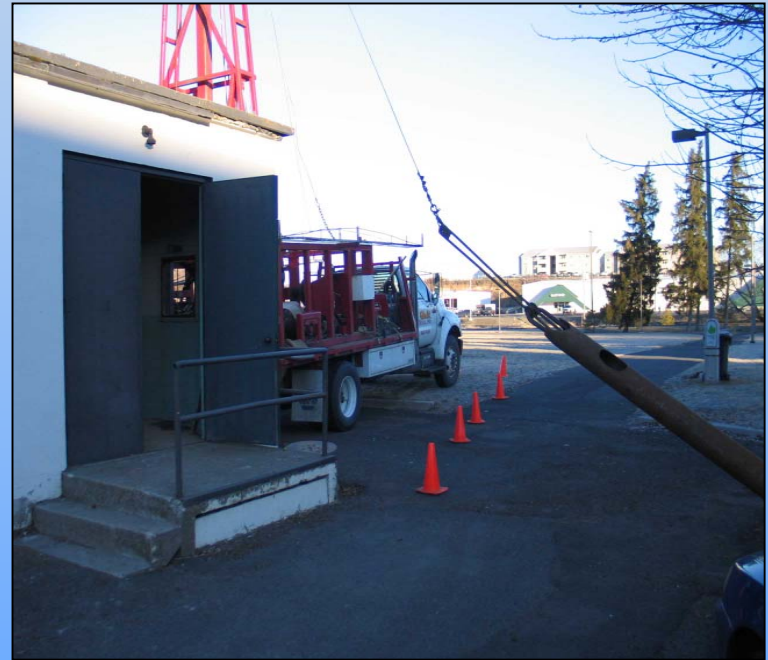
Sediment is removed with bailer
