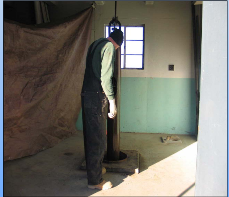
Guiding bailer in and out of well.
